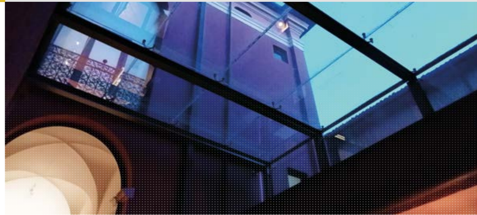
The new roofing of the internal atrium of the Busseto Library.
